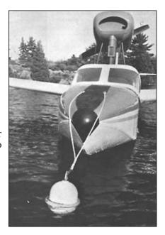
alternatives. Hulled aircraft have a single ring or cleat attached to the bow, along the center line of the aircraft. Unfortunately this is not true for the Lake. Its modest cleat is installed on the port side of the nose causing the ship to 'fishtail' in strong winds. However, anyone frequently using this method of securing the aircraft can easily install a second cleat on the opposite side of the bow.
